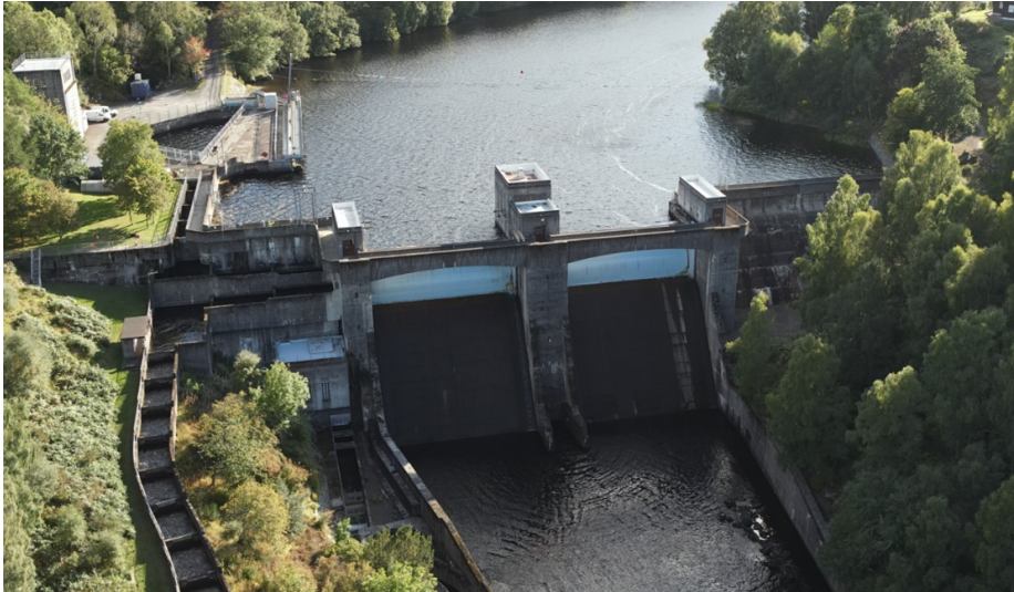
Drone view of a hydropower dam
