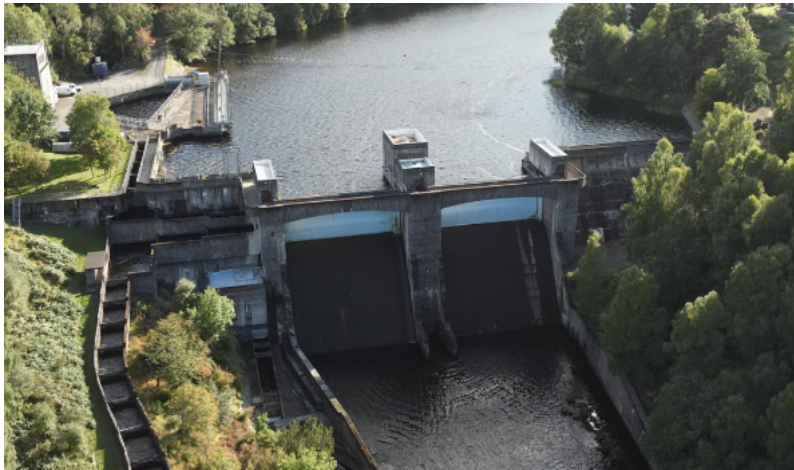
Drone view of a hydropower dam
