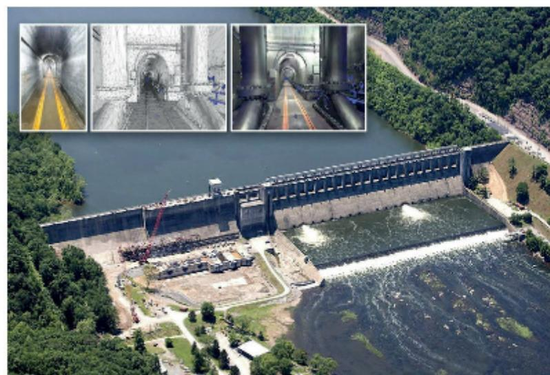
Right: As part of the process of creating digital twins of Bluestone Dam in West Virginia, researchers have created 3D models of many of the corridors and inner workings of the facility. These models move from a photograph to the creation of the geometry and wireframe, and then finally to the final color model (USACE Courtesy Photo)
