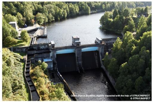
"Clunie is 72 years old and, in terms of capacity and size, the heart of a chain of power plants between Dalwhinnie, Rannoch and Pitlochry," explained Andrea Venora, head of Project Sense at Voith Hydro. "This is a gravity dam where the forces of the horizontal water pressure, the brine pressure and the mass of the structure meet.
